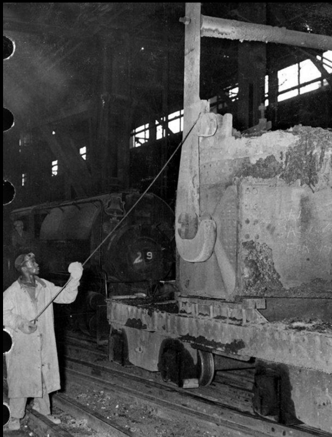
Ladle being settled into place for transportation.
